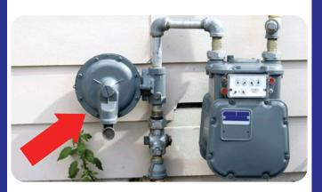
If your natural gas meter piping has a round saucer shaped piece of equipment (regulator) similar to the one on the left side of the picture above, your service may be eligible for an EFV.
